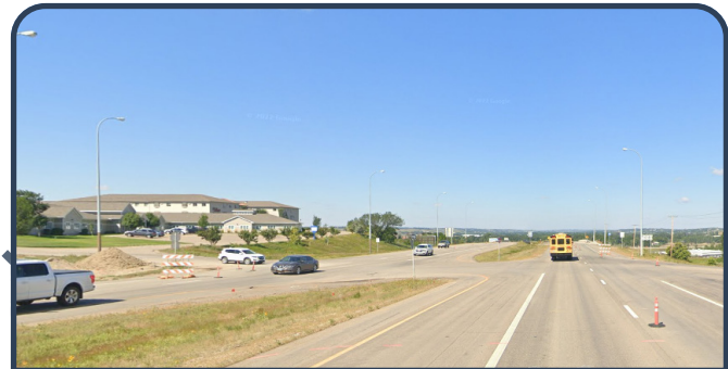
Intersection of US 2/52 and Burdick Expressway – one of the highest crash locations in the state without south access
