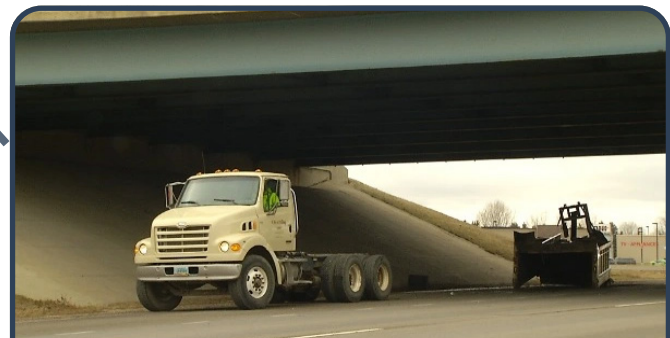
With a clearance of 16 feet, the operationally deficient 16th Street Bridge has been struck by oversize truck loads numerous times in the past decade.
