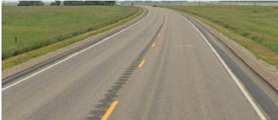
Example of both Edge and Centerline Rumble Strips on a state highway
