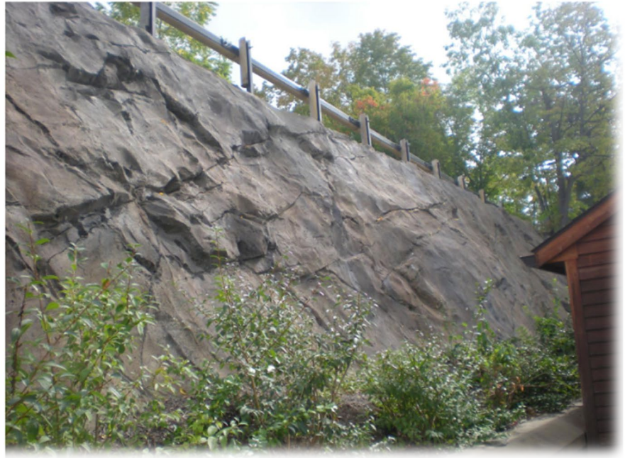
Figure 2 &3. Sculpting and stained finish of shotcrete. $$-$$$$. 4-10 extra business days depending on desired finish and done through reputable subcontractor of GSI.
